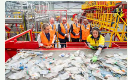
Australia's largest PET bottle recycling facility that began operation in New South Wales
