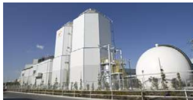
External view of Bio Energy Corporation Jonanjima Plant
