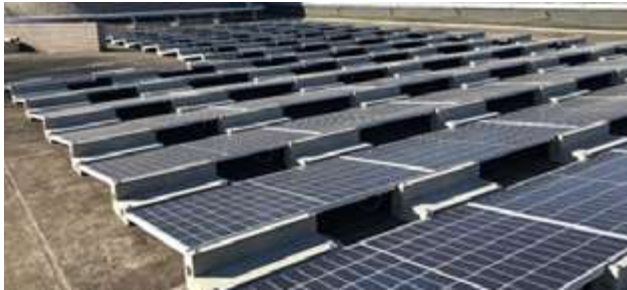
Rooftop of the Visitors' Building of Asahi Breweries, Ltd. Ibaraki Brewery
