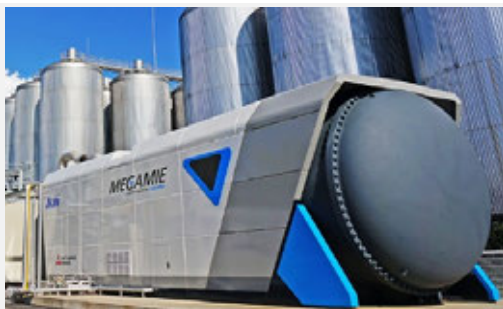
A fuel cell power generation system using biomethane gas generated from brewery wastewater
