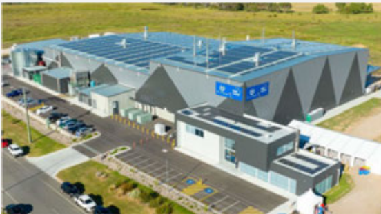
Operation of PET recycling facility
