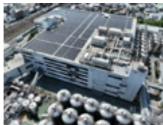
Installation of solar power generation equipment
